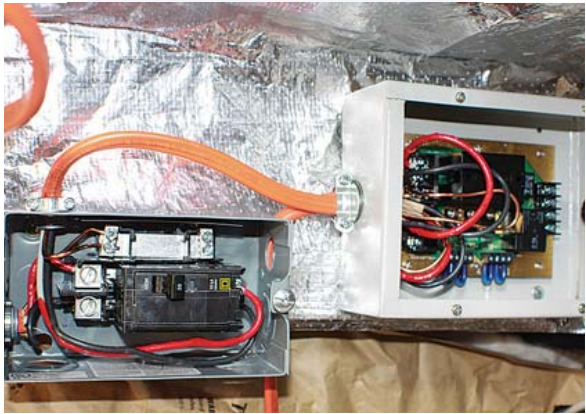
(Above, from left to right) The two circuit breakers were purchased from a local home improvement center. Before installing the Scotchlok on the air switch wire make sure the correct wire is selected. The Scotchlok connects the wire from the controller to the fan motor feed wire. It takes patience to follow the color-coded wiring diagram, but the instructions walk the installer through the process.
