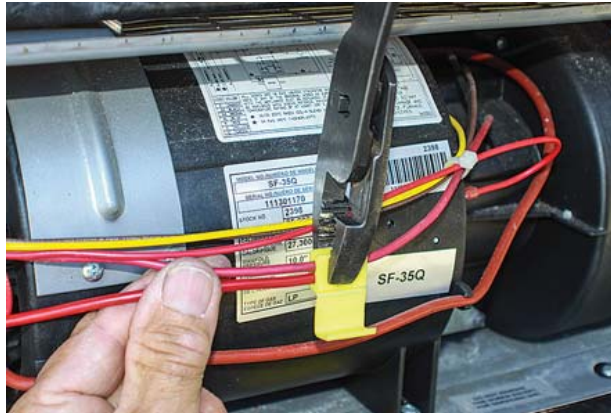
(Above, from left to right) The two circuit breakers were purchased from a local home improvement center. Before installing the Scotchlok on the air switch wire make sure the correct wire is selected. The Scotchlok connects the wire from the controller to the fan motor feed wire. It takes patience to follow the color-coded wiring diagram, but the instructions walk the installer through the process.
